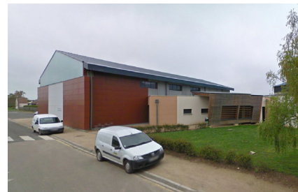
Extension du gymnase Patay (45)
