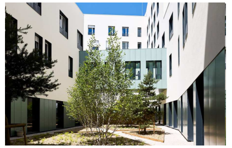
Extension centre hospitalier des Massues, Lyon 5
